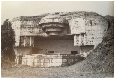
Illustration 1. An Atlantic Wall Bunker.
